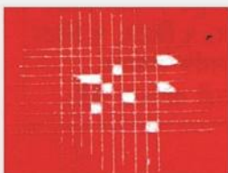
Poor Paint adhesion without application of Steel Guard Nanocoat
