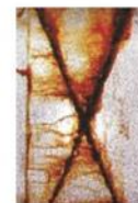
Photo of cross cut test Epoxy paint & Salt Spray after 120 hours without STEEL GUARD.
